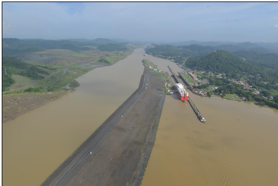
Figure 24: View of cofferdam from the south side (long term condition)
