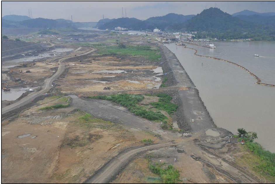
Figure 23: View of cofferdam from the south side (construction stage)
