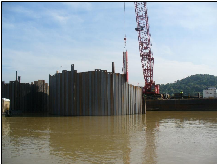
Figure 18: Driving piles in a cell by vibration
