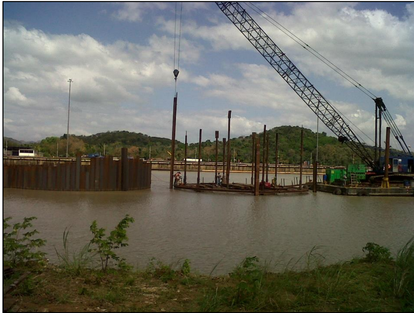
Figure 17: Template in position
