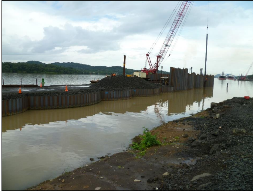
Figure 19: Filling operation of the cells
