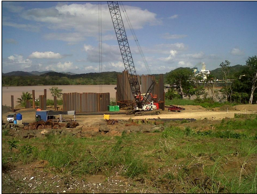
Figure 20: Landside cofferdam in the south end
