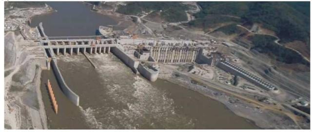
Fig. 2. General overview of progress of work as of January 2018 (photo: Marie Keller) From left to right: lock, spillway, low level outlet, intermediate block, power house and fish facilities
