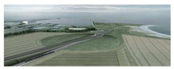
Figure 8. Tunnel portal on Fehmarn. The elevated landscape was retained. No larger revetment was necessary like on the Danish side. (see Figure 9)
