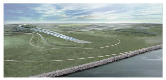
Figure 9. View of the portal area at Lolland protected by a revetment
