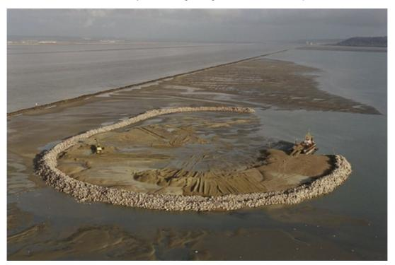
Figure 4. Bird Island constructed using dredged sediment.
