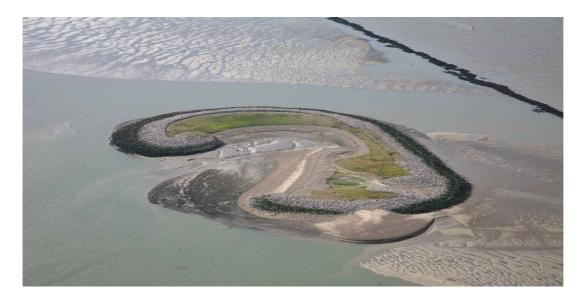
Globally the project reused 26 MM m³ sediment, of the total 45 MM m³ dredged for the new channel and basin.
