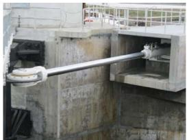
Fig. 9: Large Cylinder operating a miter gate
