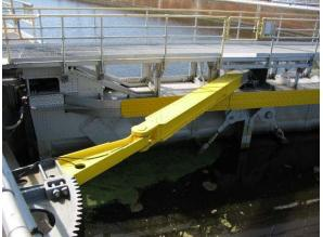
Fig. 14: Miter Gate Strut Assembly
