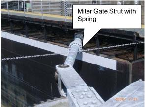
Fig. 13: Miter Gate Strut Spring
