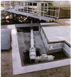
Fig. 7: Mechanical Linear Drive at a Miter Gate
