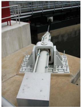
Fig. 4: Direct Connected Miter Gate Cylinder
