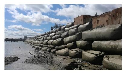
Figure 13: Geotextile megabags retaining wall
