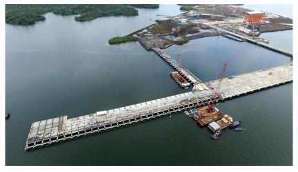
Figure 2: Wharf and trestle under construction. Progress 80%
