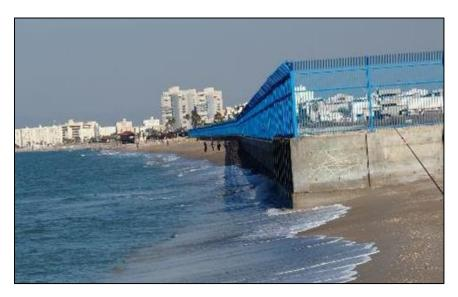
Figure 27: Beach width In front of concrete fence before sand nourishment
