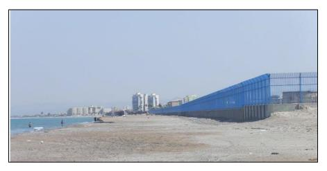
Figure 28: Beach width In front of concrete fence after sand nourishment
