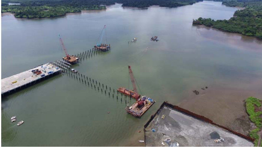
Figure 16. Bulk-Handling Wharf Construction
