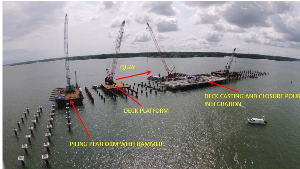
Figure 15. Top-Down Container Quay Construction
