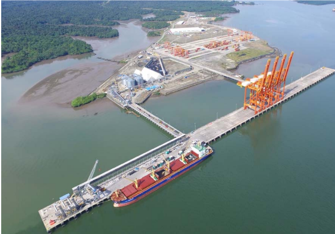
Figure 20. Completed Container- and Bulk-Handling Wharves
