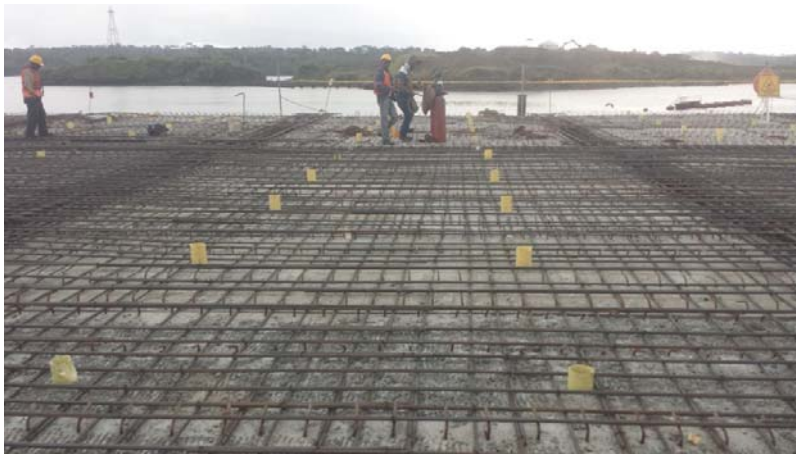
Figure 19. Sequential Deck Construction
