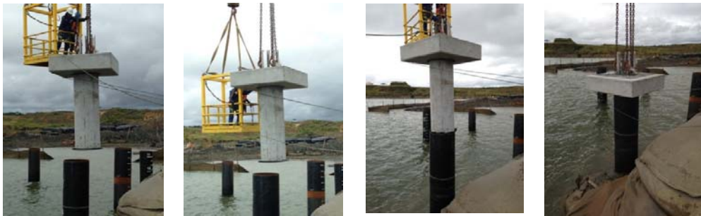
Figure 18. PC Pile Plug Installation
