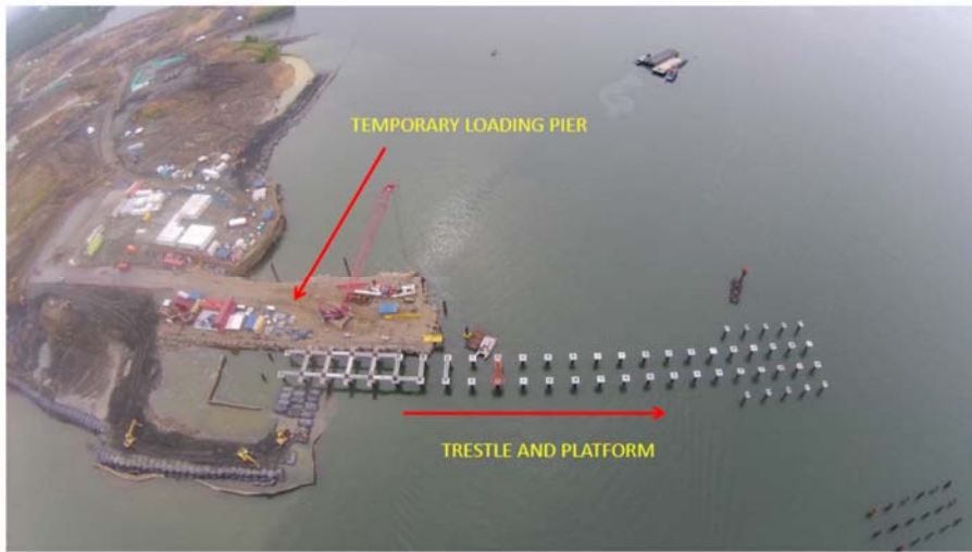
Figure 17. Container Trestle Construction
