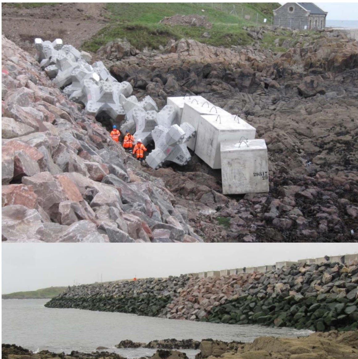
Figure 14: North breakwater under construction
