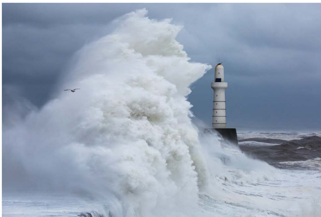
Figure 6 Wave condition at the existing South Breakwater, Aberdeen Harbour 7 January 2016
