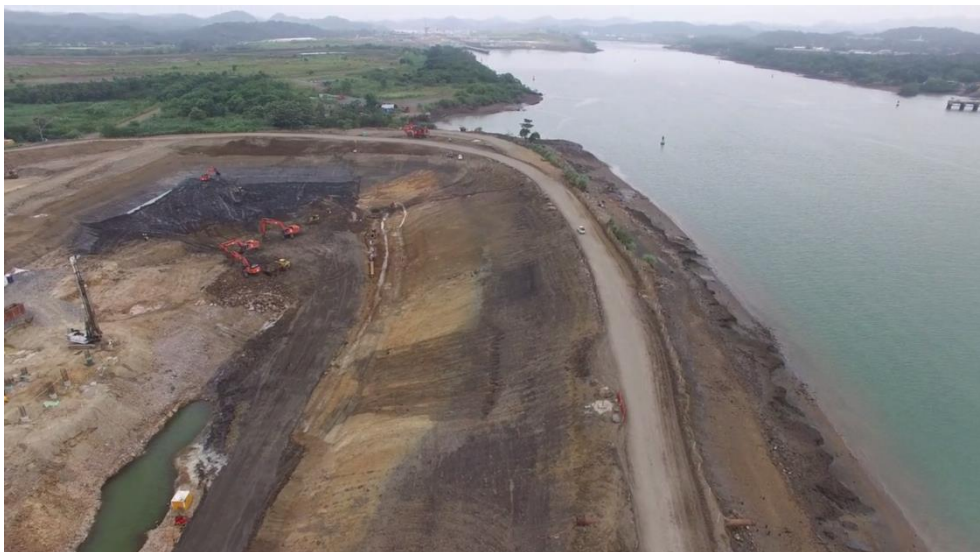
Figure 10: Dry excavation works
