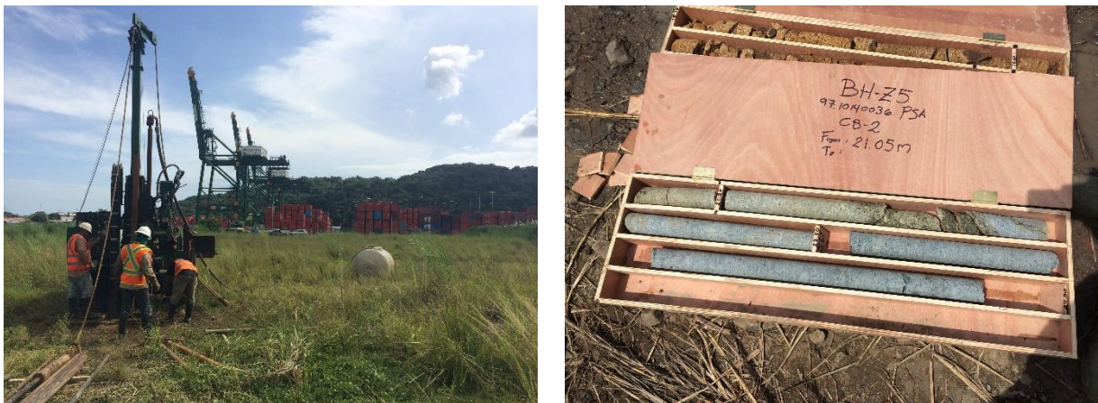
Figure 8: Borehole Drilling and Typical Core Box
