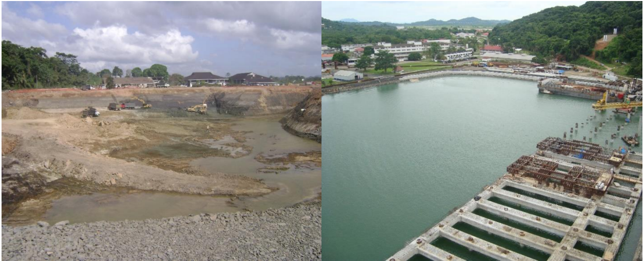
Figure 3: Phase 1 Quay Deck Construction
