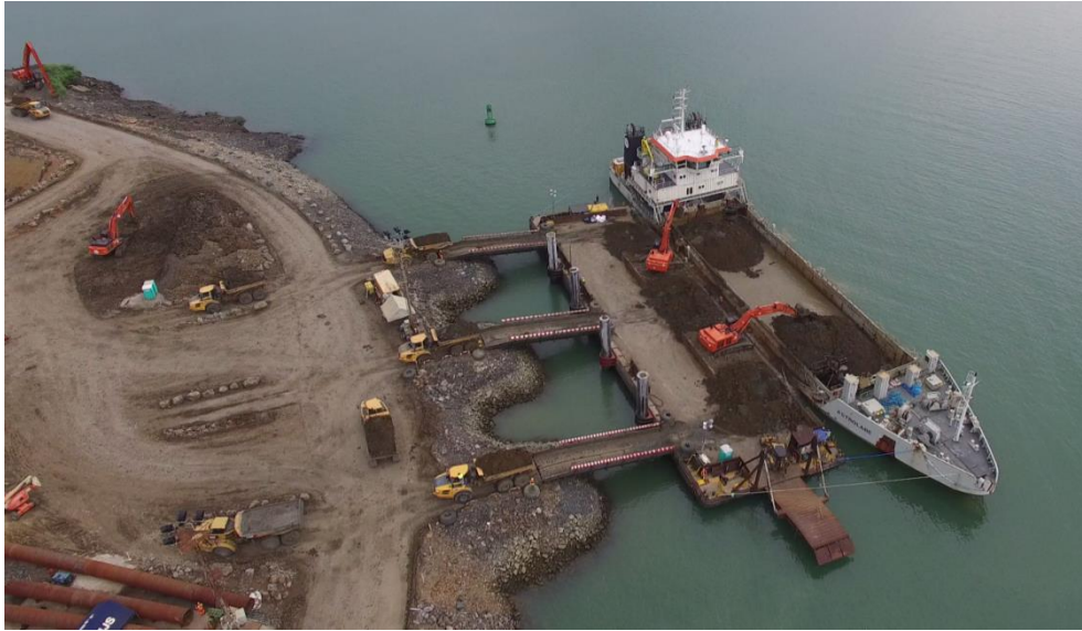
Figure 9: Temporary loading facility for off-shore disposal
