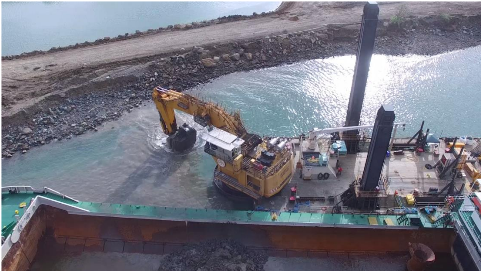
Figure 13: Dredging of loose upper layer with backhoe dredge
