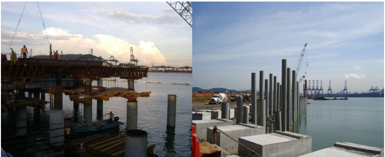
Figure 4: Phase 1 Quay Deck Construction
