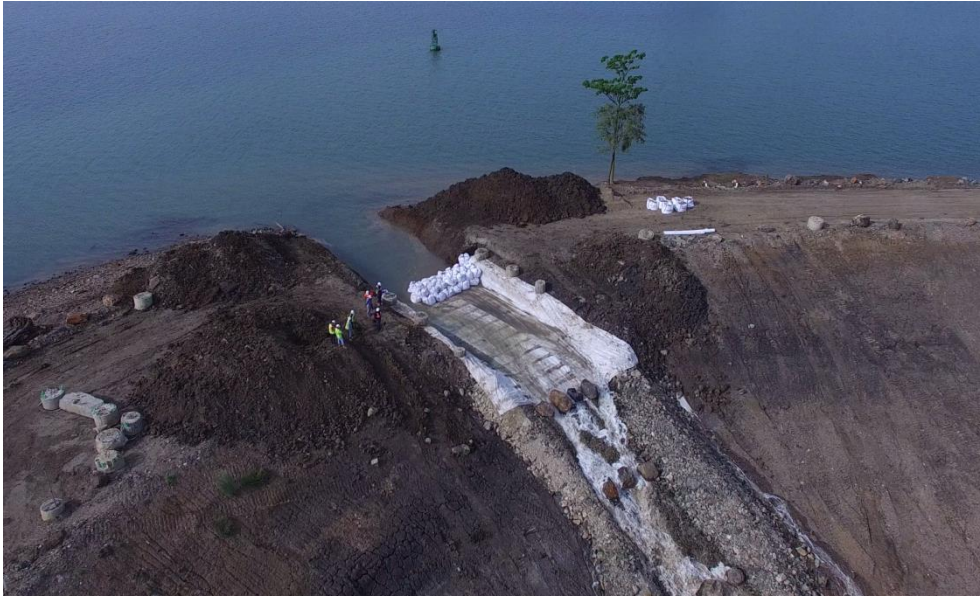
Figure 11: Controlled start of flooding
