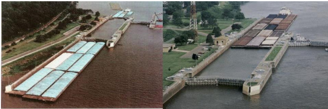
Figure 2: Multiple locking of a pushed convoy in the USA
