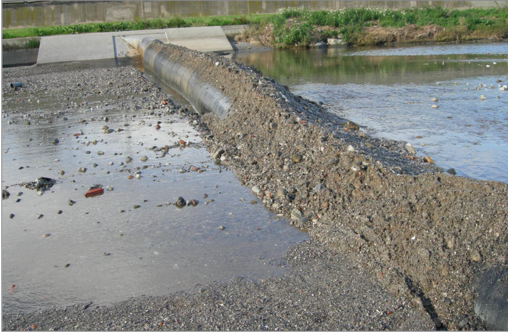
Figure 2: An air-inflated rubber gate with sediment (courtesy of Dyrhoff Ltd.)
