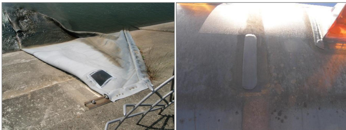
Figure 4: Repair Patches on a rubber membrane
