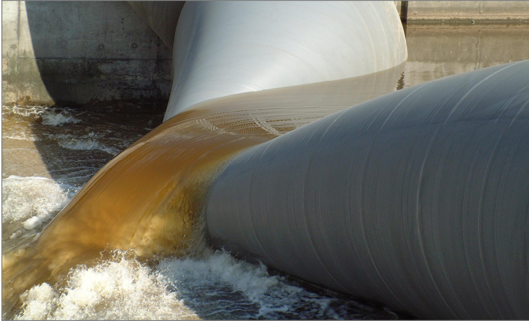
Figure 8: V-notch with an air-filled rubber gate
