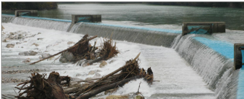
Figure 1: Situation with non-perpendicular flow and (limited) overflow
