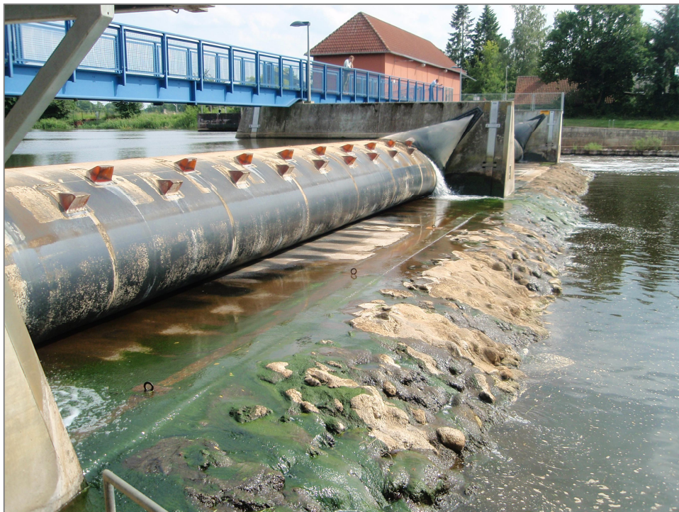
Figure 1: Weir Marklendorf - first inflatable gate at German Waterways
