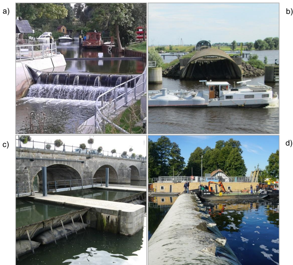
Figure 2: Applications of inflatable gates at waterways
