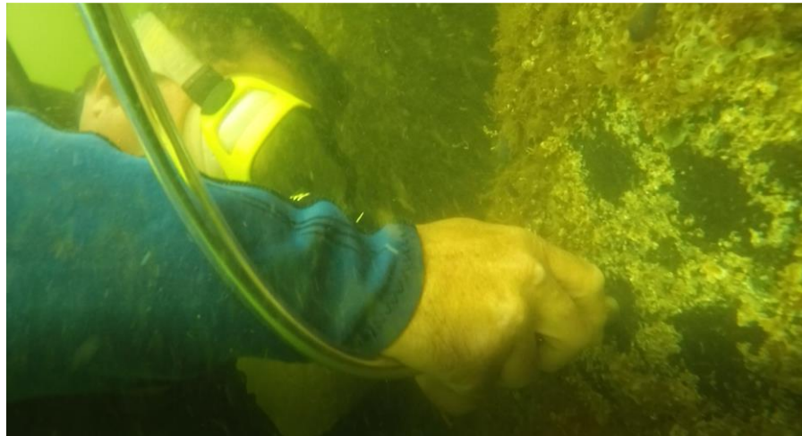
Fig. 13 Example of thickness measurement at Caldera sheet-pile wall, 2017.
