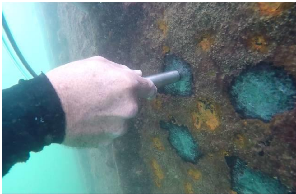
Fig. 3 Underwater Procedures at the Marina in Quepos (Above) Cleaning of measurement points (Below) Thicknesses measurement with ultrasonic sensor.
