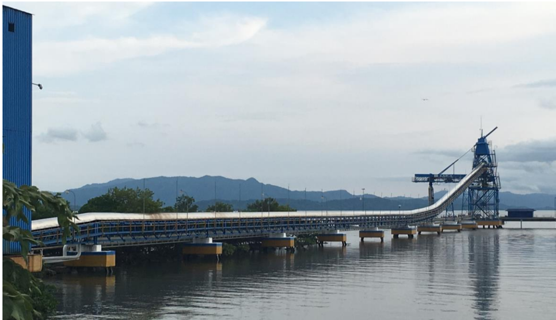
Fig. 17 Punta Morales Pier (Above) Layout of the pier including Charging Platform, Berthing Dolphins and Conveyor supports (Below) General View of Trestle Supports from land.
