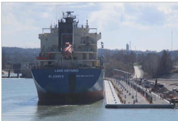
Photo 1: Completed Tie-Up Wall Construction
