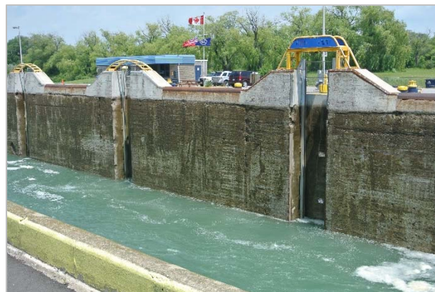
Photo 2: HFM System in Lock
