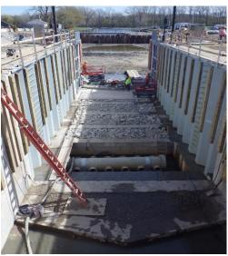
Figure 3: Diffuser System in Extended Lock Floor
