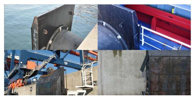
Figure 3: Damaged fender panels at Euromax Container Terminal Rotterdam (Photos PoR)
